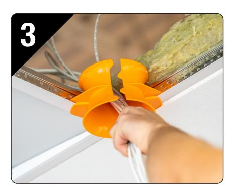
3. With the ceiling grid slotted between the Cable Funnel's tabs, push until the Cable Funnel locks into the corner. You are now ready to run your wires!
