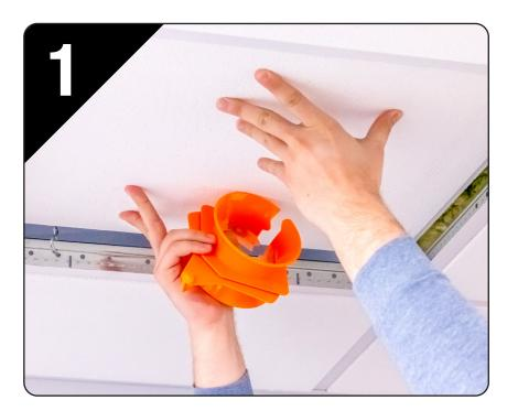
1. To protect ceiling tiles from damage, remove both tiles in the corner of the ceiling you wish to install the Cable Funnel. Then position the Cable Funnel finger loop down as shown.
